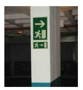
Standard rectangular Type 1 signs often do not suit installation onto pillars due to their shape and a reduced effective viewing distance due to their relative size. Evacuation signs specifically developed for pillars allow pictograms to be larger, therefore providing a greater viewing distance. The image shown illustrates the comparison between the two types of evacuation signs and the pictogram size.
