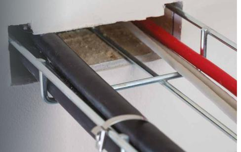
Abbot Fire Group's trained technicians will assess the area, and carry out the relevant remedial action using intumescent materials. This can include using acoustic intumescent sealant where noise between compartmentations needs to be kept to a minimum.
